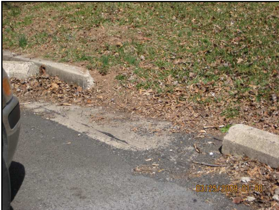
Photo 4 Curbing Removed to Facilitate Drainage during Hurricane Floyd Located on the Northern Portion of the Property Near 403 Skyhawk Drive
