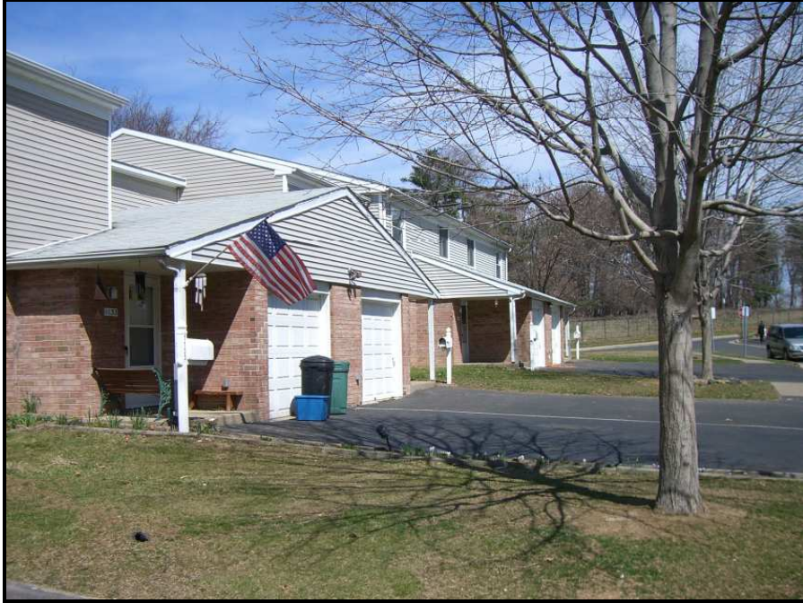
Photo 1 Typical Shenandoah Woods Housing Unit
