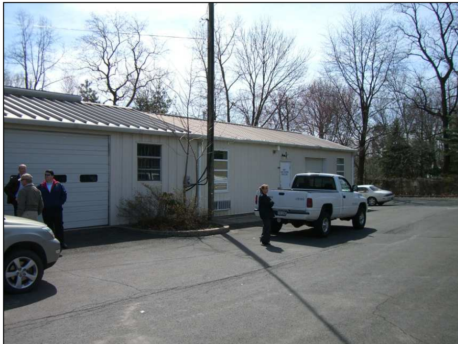
Photo 6 Shenandoah Woods Housing Maintenance Building
