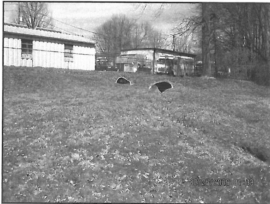
Photo 4 Stormwater Retention Pond Located South of Facilities Maintenance Department Garage
