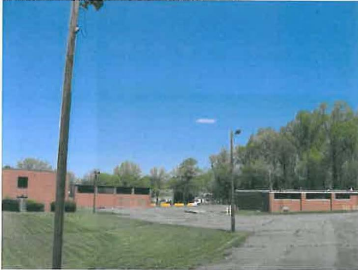
Figure 1. Overview of the building layout and asphalt surfaces at the Horsham Memorial USARC, facing north (from left: main block of the administration building; center: rear drill/assembly hall wing; and right: OMS)
