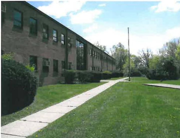
Figure 2. Main (West) Elevation of the Horsham Memorial USARC, facing Southeast, showing original brick veneer exterior and metal and glass assembly at main entrance
