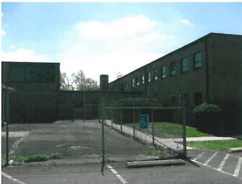
Figure 4. North Elevation of the Horsham Memorial USARC facing south, showing rear of the main block, one-story hyphen, and double height rear wing with clerestory lights for the drill/assembly hall facing south
