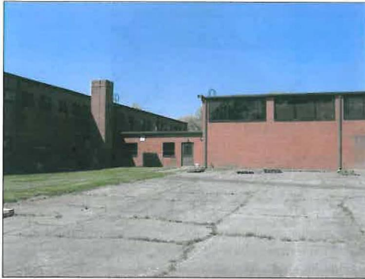
Figure 9. South elevation of the Horsham Memorial USARC, showing rear of the main block, one-story hyphen, and double-height rear wing with clerestory lights for the drill/assembly hall, facing northwest.
