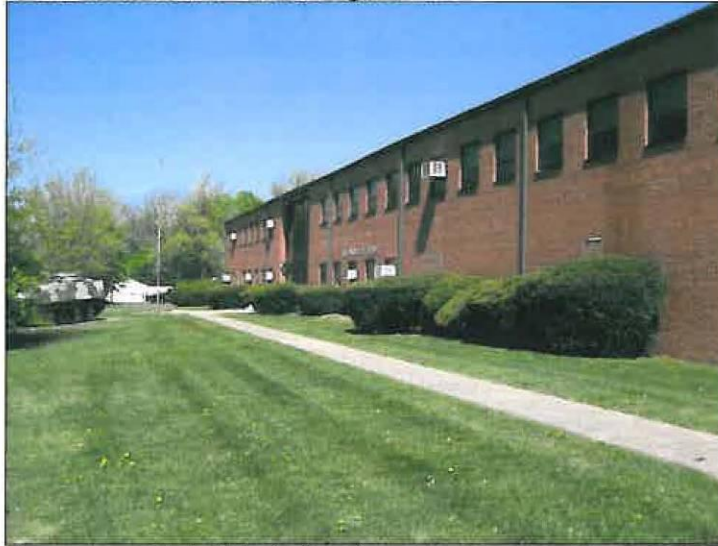
Figure 1. Main (West) Elevation of the Horsham Memorial USARC, facing Northeast, showing original brick veneer exterior with infilling of original openings.
