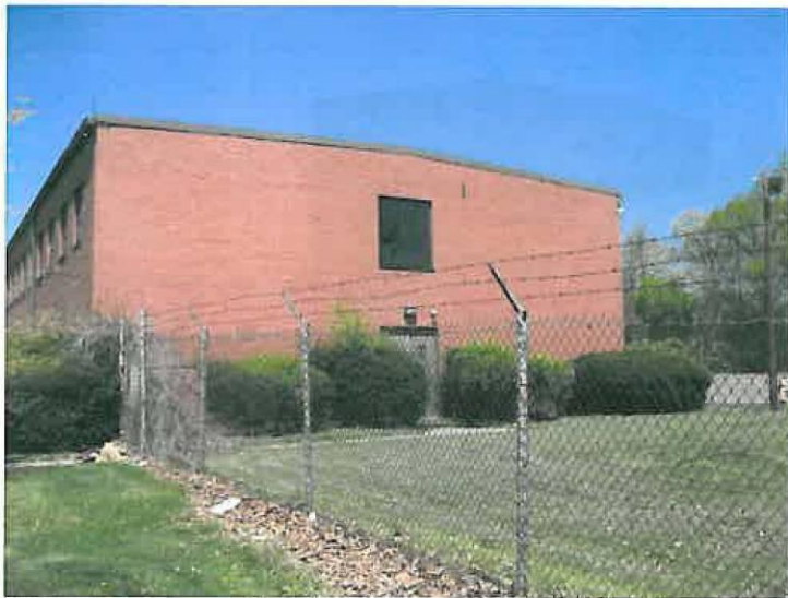
Figure 6. South Elevation of the main block of the Horsham Memorial USARC, facing north
