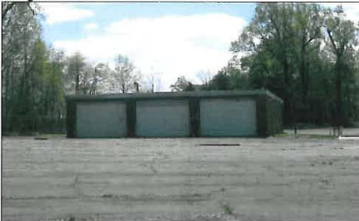
Figure 8. Main elevation of the Organizational Maintenance Shop (OMS), facing south, located southeast of the Main building at the Horsham Memorial USARC.
