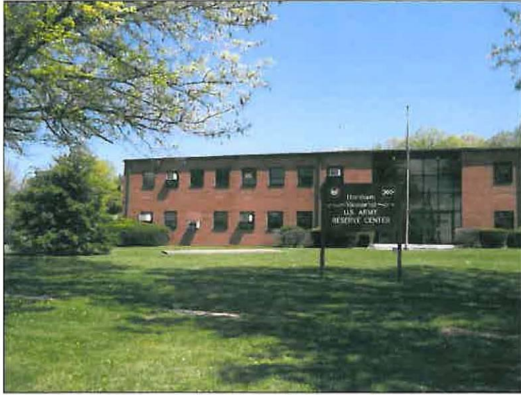
Figure 9. North end of the Main (West) Elevation of the Horsham Memorial USARC, facing East, showing glass and metal assembly at main entrance and brick infilling of former openings for a window and several vents.
