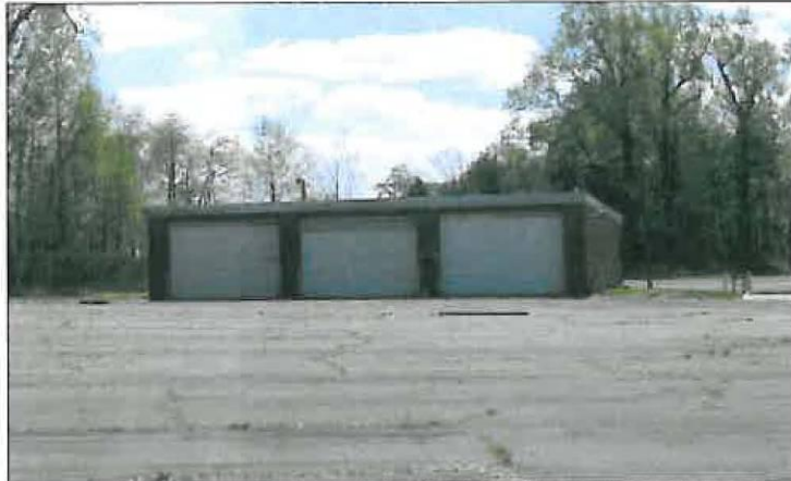
Figure 11. Main elevation of the Organizational Maintenance Shop (OMS), facing south, located southeast of the Main building at the Horsham Memorial USARC.
