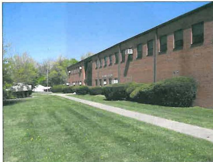
Figure 4. Main (West) Elevation of the Horsham Memorial USARC, facing northeast, showing original brick veneer exterior with infilling of original openings, affixed signage, flagpole, and concrete pad for vehicle display.
