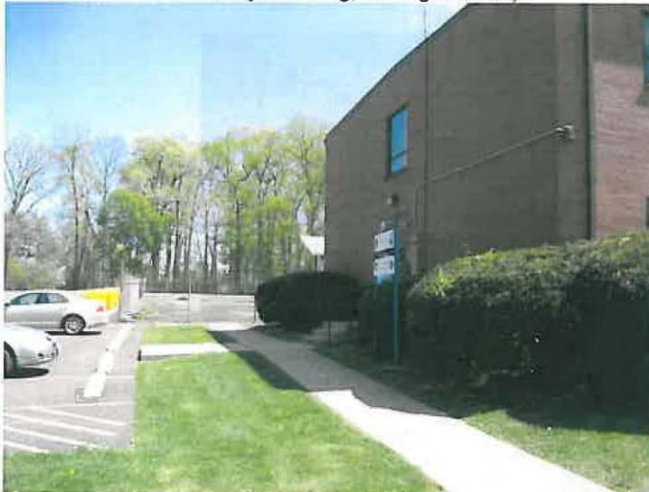
Figure 2. North elevation of the main block of the Horsham Memorial USARC facing east, showing side-gable roof, walkways, parking and signage.
