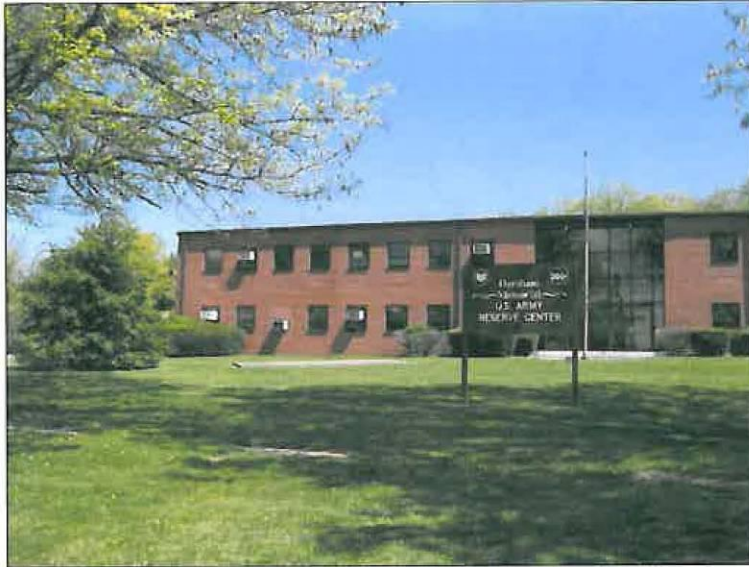
Figure 3. North end of the Main (West) Elevation of the Horsham Memorial USARC, facing east, showing glass and metal assembly at main entrance, brick infilling of former openings for a window and several vents, signage, and flagpole.
