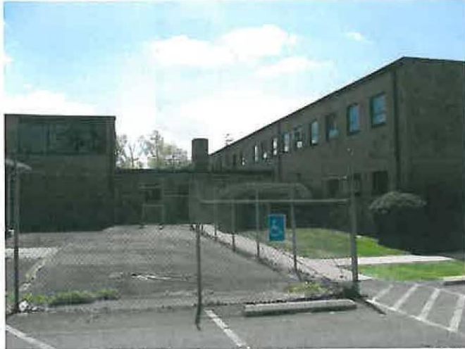
Figure 7. North Elevation of the Horsham Memorial USARC facing south, showing rear of the main block, one-story hyphen, and double height rear wing with clerestory lights for the drill/assembly hall facing south
