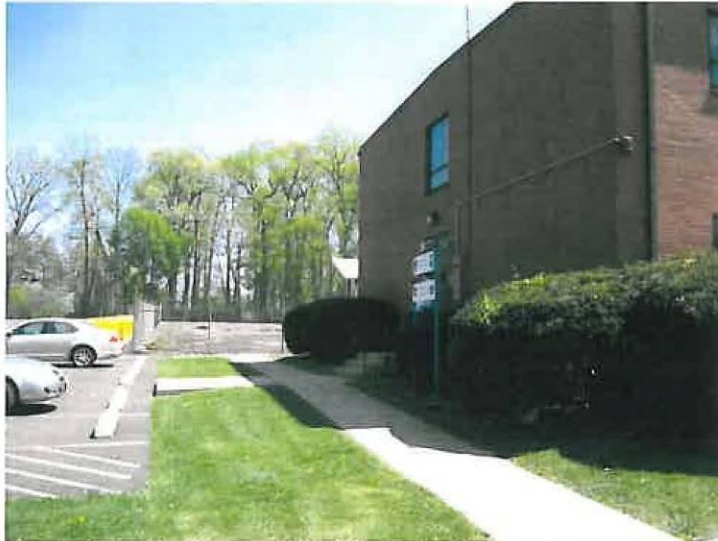
Figure 3. North elevation of the main block of the Horsham Memorial USARC facing east.
