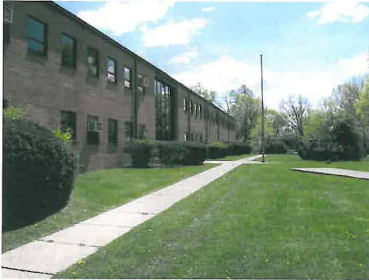
Figure 5. Main (West) Elevation of the Horsham Memorial USARC, facing southeast, showing original brick veneer exterior, metal and glass assembly at main entrance, flagpole, and concrete pads for vehicle display.
