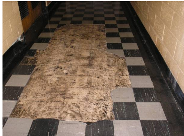
10. Floor tiles with ACM in the main building.
