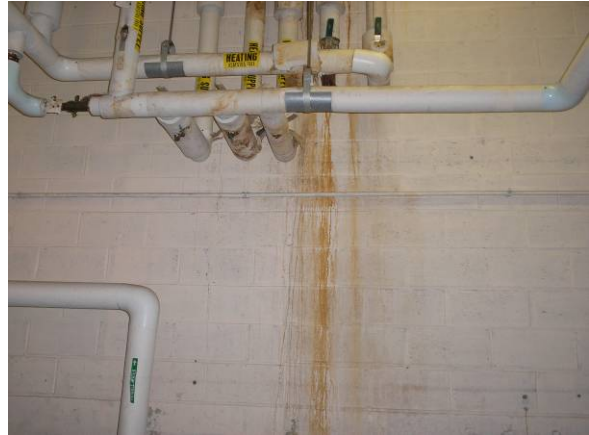
2. Boiler room inside the main building, facing west.
