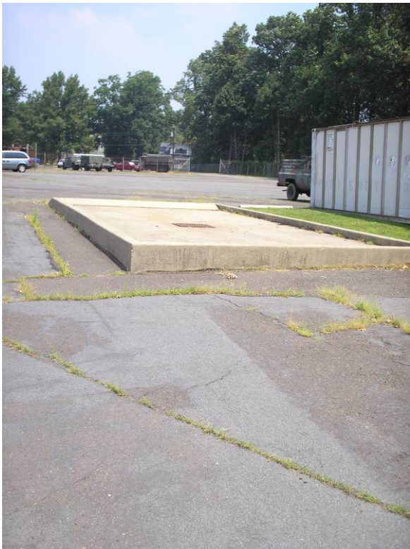
3. Wash rack, west side of OMS building.
