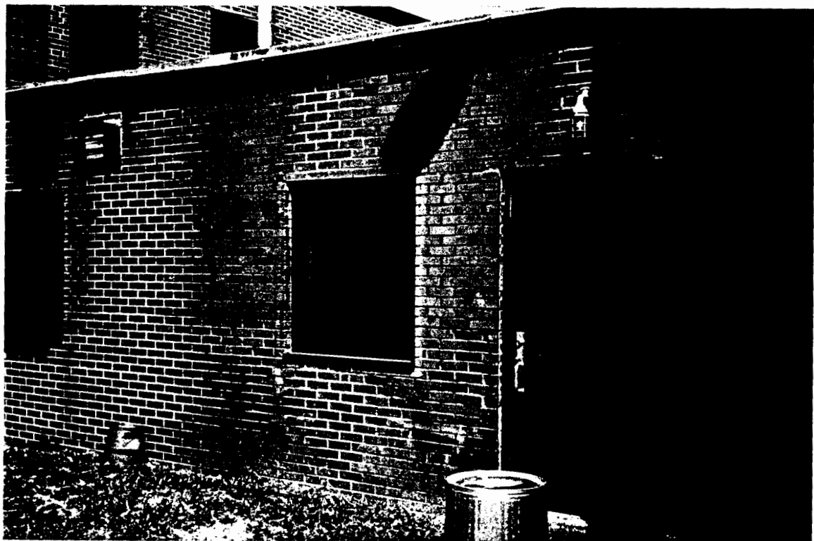
Photo 6: Repointing, south side of USAR Center by drill hall
