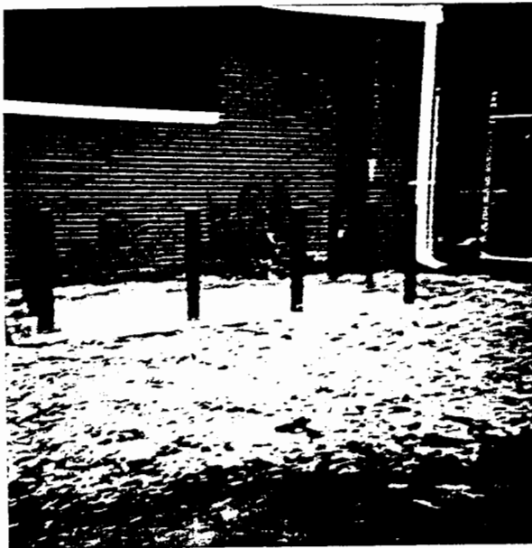
JUNE 1996-CONCRETE PAD WITH BOLLARDS
